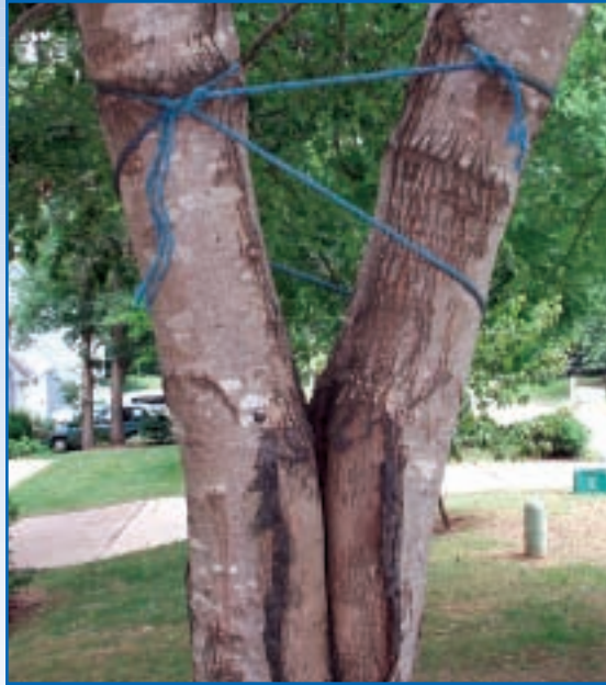
After a hurricane ten years ago, the home owner managed the split with rope and pruning paint. Now the rope is swallowed, creating a new risk of failure.
