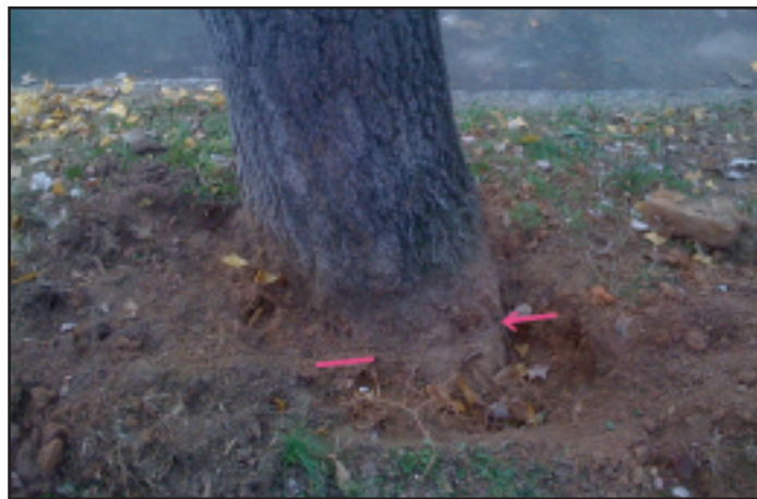
Human error causes instability issues. Burying the trunk flare resulted in a stem-girdling root. Removing the root, and the fill, dries the root crown and restores safer conditions.
