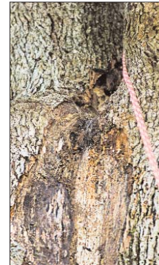
Andersonville — Wound at main fork of landmark post oak. No callus growth in five years, decay advancing, root damage increasing, high target rating; fatal damage from lightning strike. Courtesy Chip Hillreth, ArborCarolina
